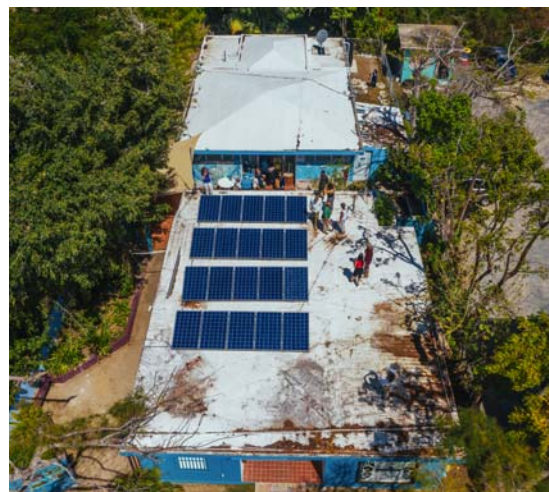
Solar panels, Community center.
